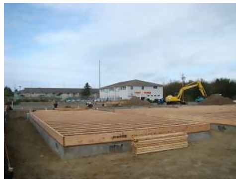
Front view of Unit #A.
