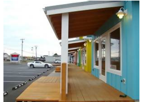
The Boardwalk along the front shops.
