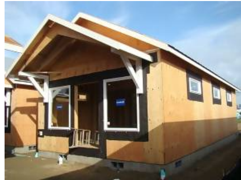
Rear view of Unit #A (Boardwalk side).
