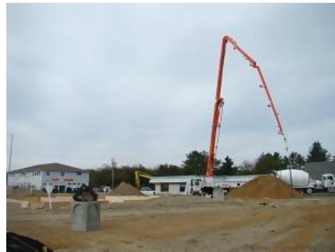
Concrete being poured for the stem walls.
