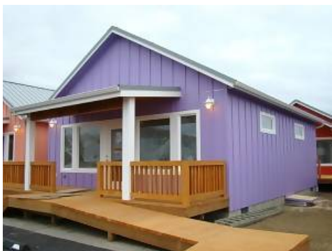
Front view of Unit #G (Minard Ave side).
