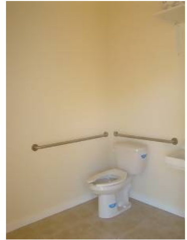
Unit #A ~ Handicap Accessible Bathroom.
