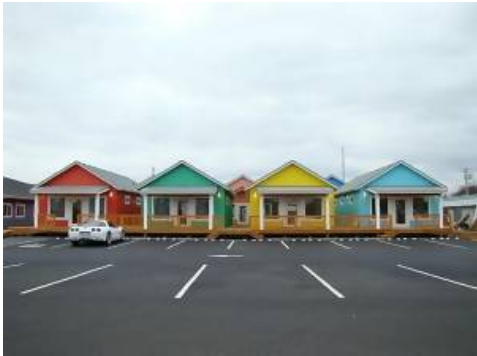
View of the Shops that front Pt Brown Ave w/ a paved parking lot.
