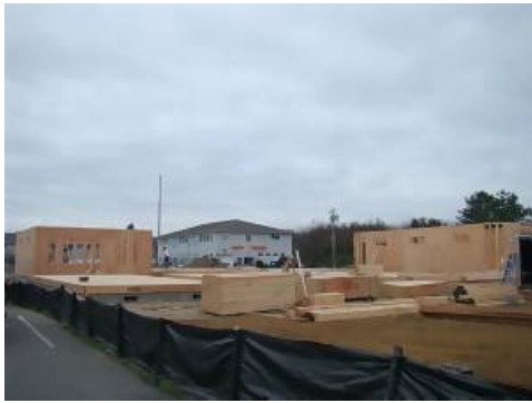
Front view of the Shops that front Pt Brown Ave.
