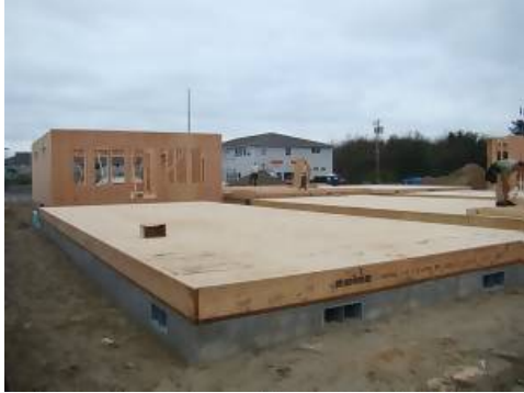
Front view of Unit #A.
