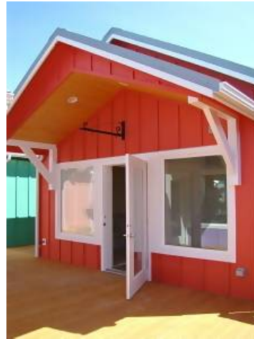
Rear view of Unit #A (Boardwalk side).
