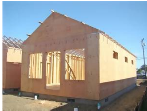
Rear view of Unit #A (Boardwalk side).
