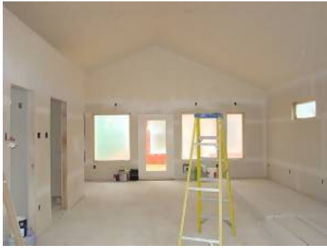
Interior view of Unit #G ~ looking towards the boardwalk entrance.
