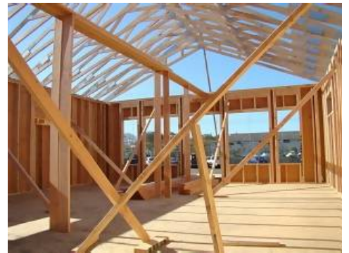
Interior view of Unit #E ~ looking towards the front entrance.
