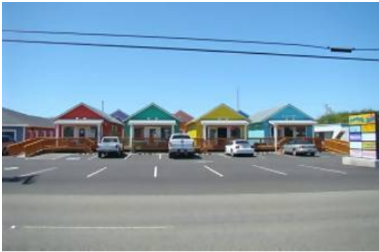
The front Shops along Pt Brown Ave.
