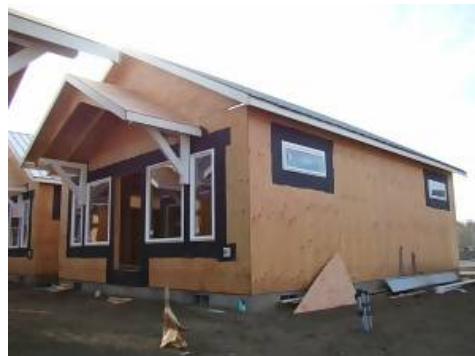
Rear view of Unit #E (Boardwalk side).
