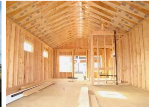
Interior view of Unit #A ~ looking towards the boardwalk entrance.
