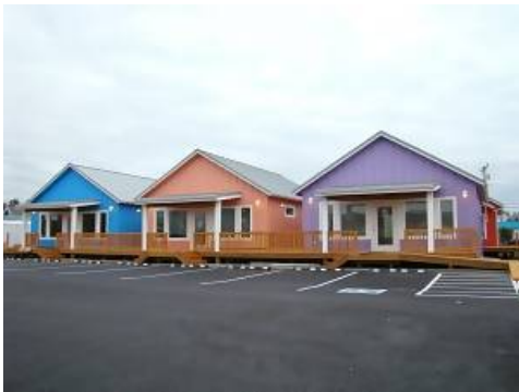
View of the Shops that front Minard Ave w/ a paved parking lot.
