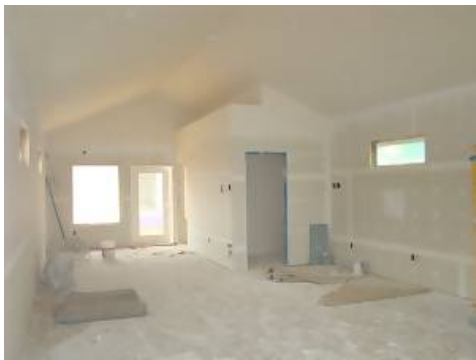
Interior view of Unit #A ~ looking towards the boardwalk entrance.
