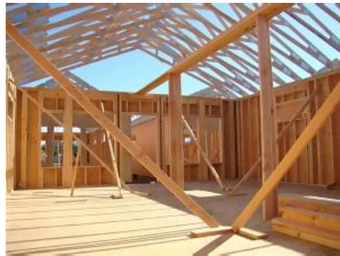
Interior view of Unit #E ~ looking towards the boardwalk entrance.
