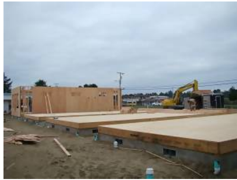
Rear view of the Shops that front Pt Brown Ave.
