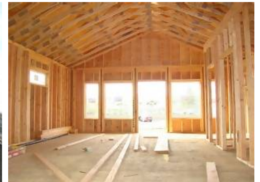
Interior view of Unit #E ~ looking towards the front entrance.
