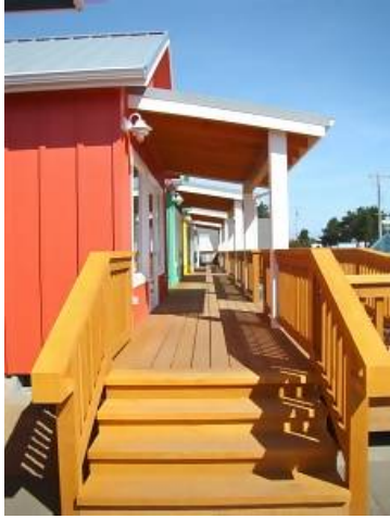
The Boardwalk along the front Shops.
