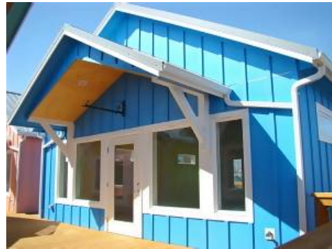
Rear view of Unit #E (Boardwalk side).
