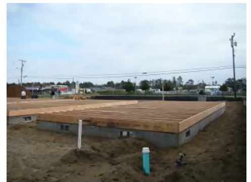
Back view of Unit #A.
