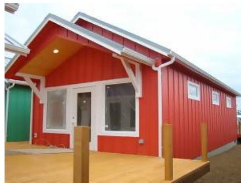
Rear view of Unit #A (Boardwalk side).
