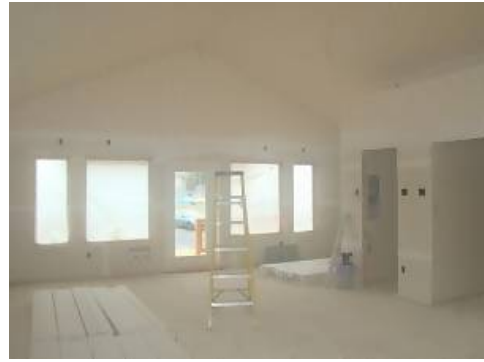
Interior view of Unit #G ~ looking towards the front entrance.
